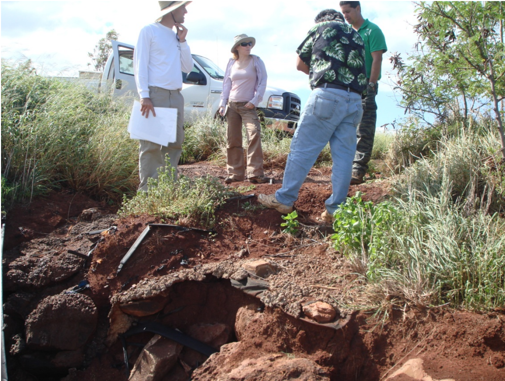
HA8: Honokōwai Structure #8; Concrete Outlet Control Structure With Horizontal Outlet Debris Ports Visible
