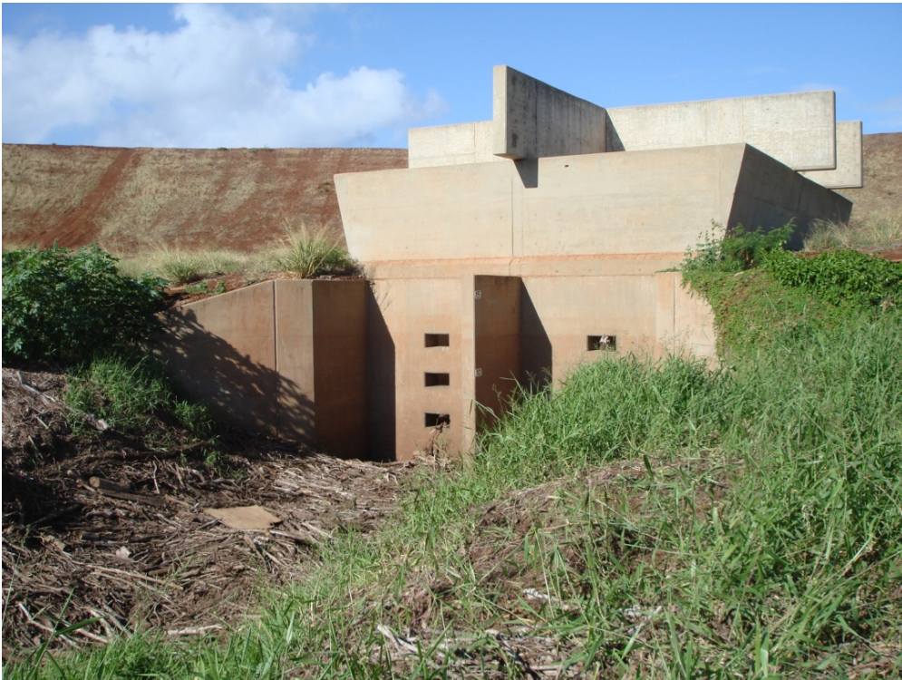
HA8: Honokōwai Structure #8; Concrete Outlet Control Structure With Horizontal Outlet Debris Ports Visible
