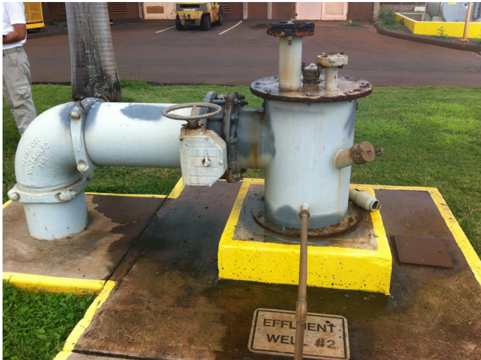
HU4: Lahaina Wastewater Reclamation Facility, Injection Well # 2
