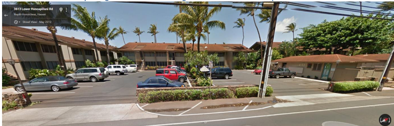
Runoff from the Hale Kai parking lot flows down to the gutter line on Lower Honoapiilani Rd.
