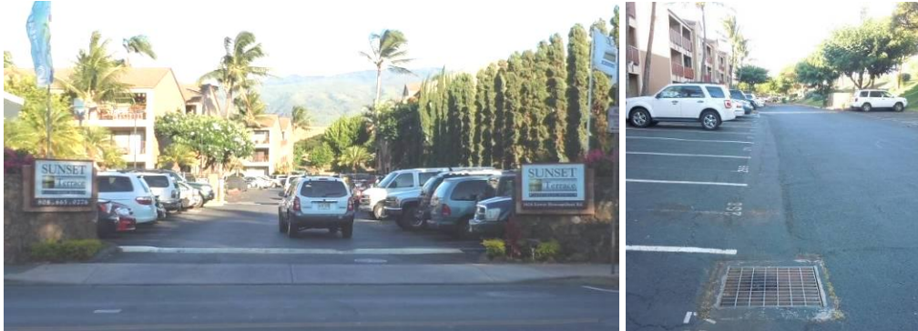
Driveway entrance to Sunset Terrace (left); catch basin in back parking area (right).
