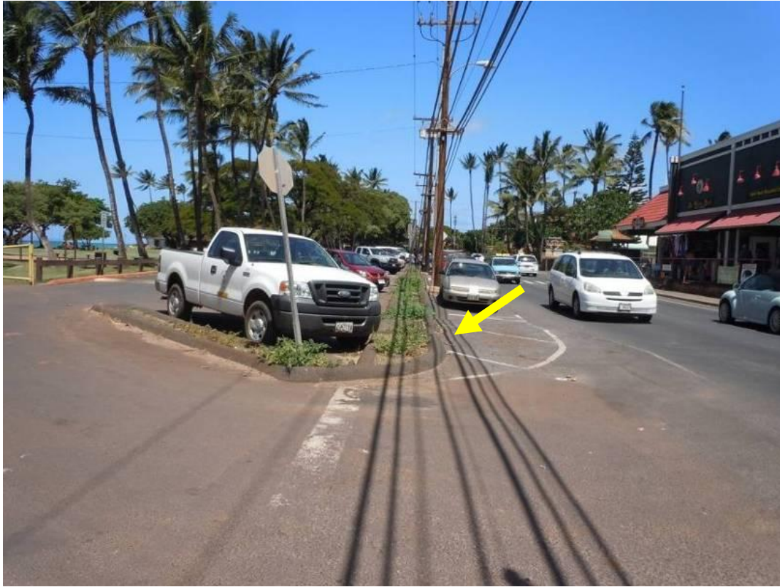
Looking north at the existing island between HBP and Lower Honoapiilani Rd, with the existing catch basin identified with the yellow arrow (top). Graphic rendering of tree trench and flow paths (bottom).
