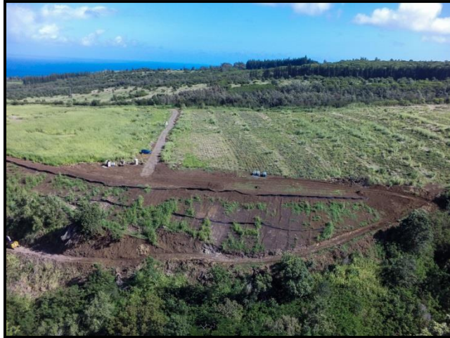
Figure 6: Cleared gulch shoulder in preparation for solar farm
